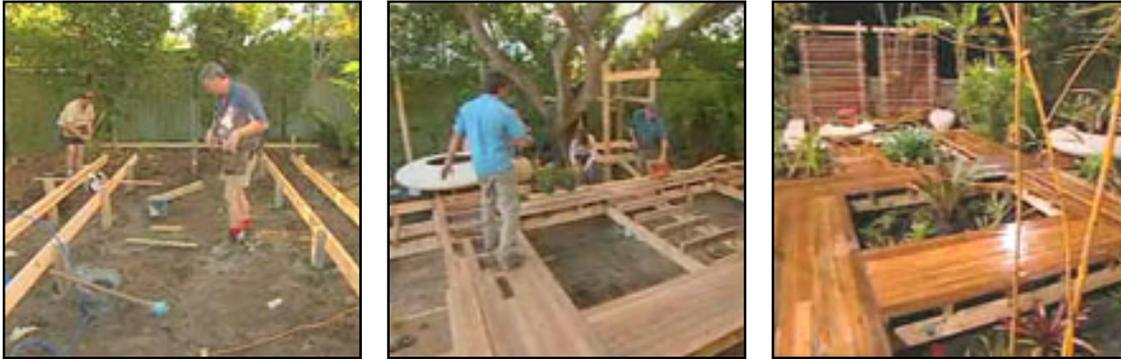
**Screens:** Jamie built decorative screens in the garden. He marked out screen locations and located post positions. H4 treated pine posts were concreted in ground using a spirit level to ensure each post was exactly vertical. Jamie then attached two lengths of rope to the top of each post and wove the rope around decking boards creating a venetian blind effect. The end of each rope was then secured to the ground.
